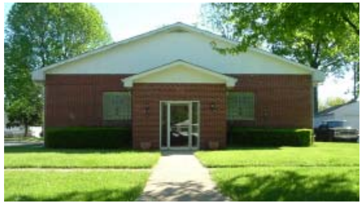
The building on Anderson Avenue before the work begins.
